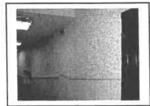
^Auditorium wall acoustical plaster.
