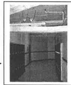
^ Non-asbestos TSI in hall >
